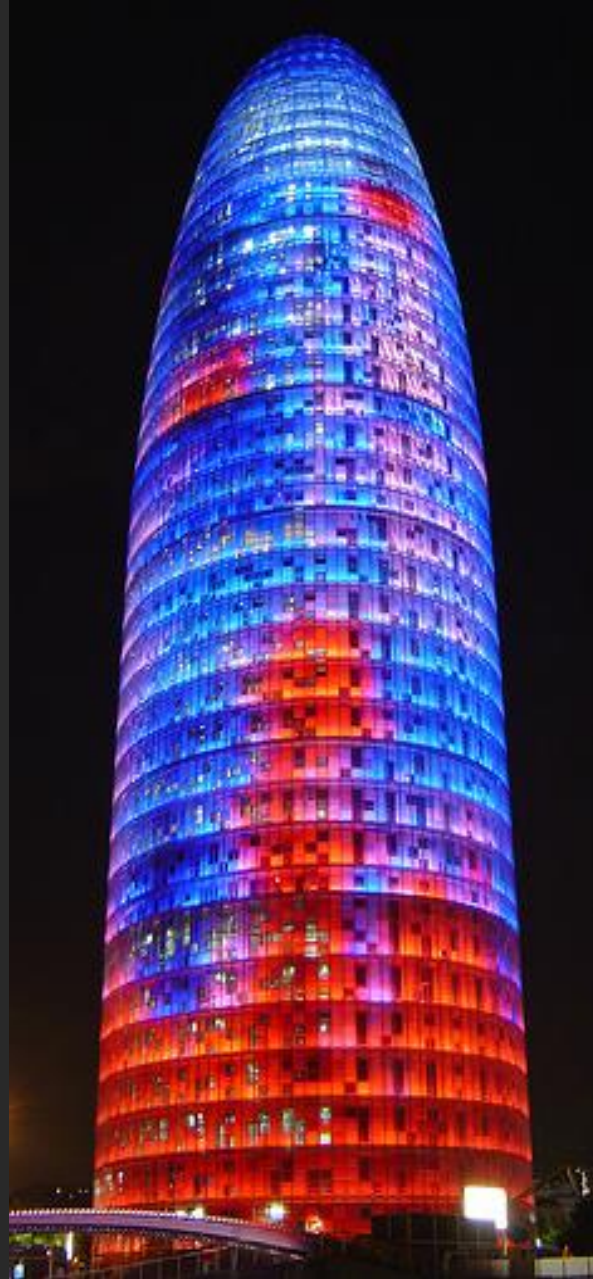
TORRE AGBAR – 2005 – ARQ. JEAN NOUVEL
